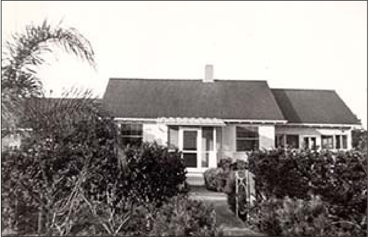
The new owners of the property are restoring the guest cottage to its original look, with Dade County pine on the floors and bead board on the walls.
